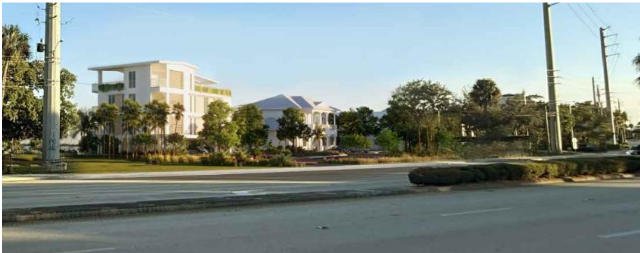
Figure 1: View of proposed building from N. Alternate A1A looking to the southeast.
