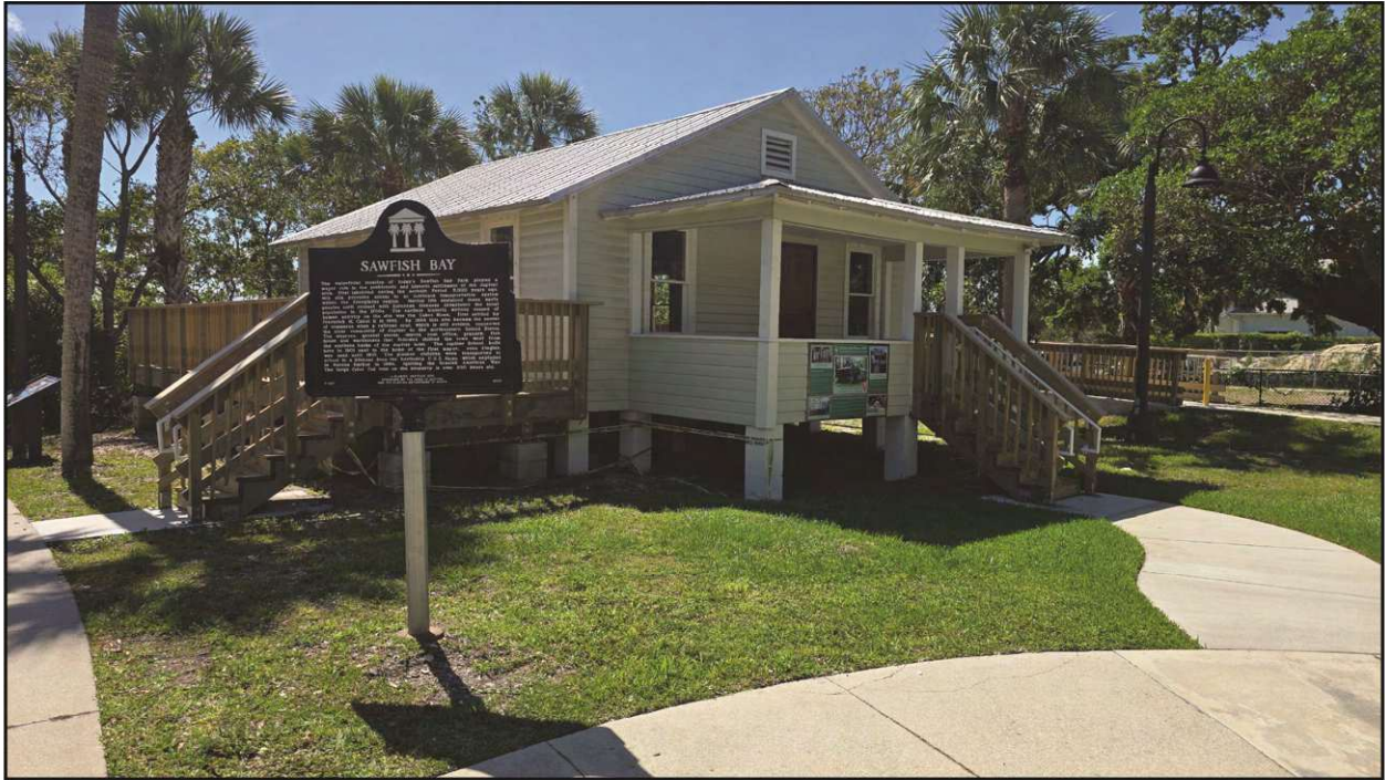
Current photograph (2026) view southeast at the Aicher House.
