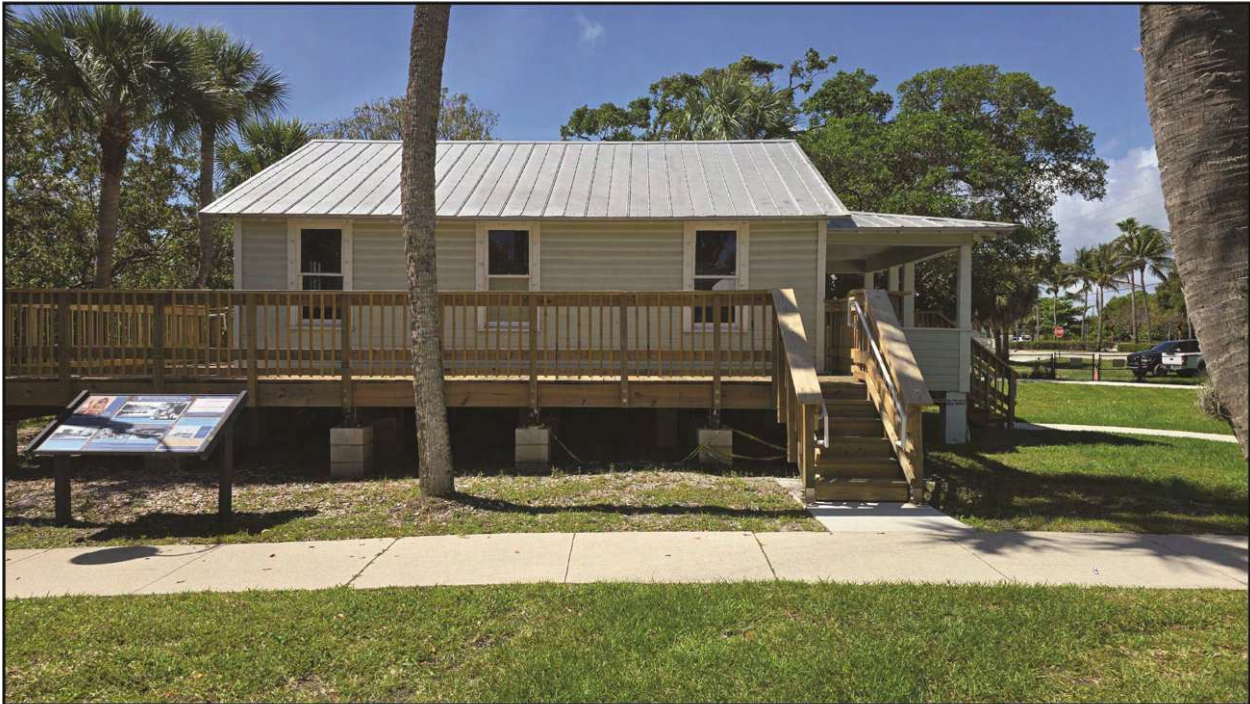
Figure 13. Current photograph (2026) view southwest at the Aicher House.
