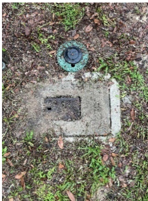
Photos of non-traffic antenna boxes taken during the Town of Jupiter pilot that proved to be a success after extensive testing in the Town of Jupiter.
