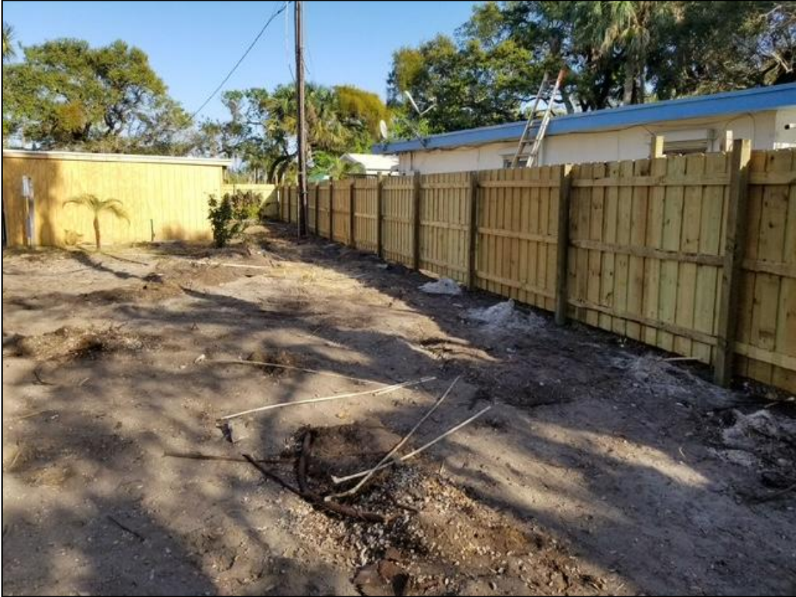
Figure 21. Post-site fill and fence installation, facing north-northwest.
