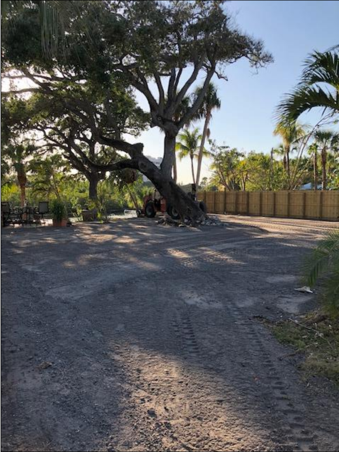
Figure 23. Post-fence installation and site dirt fill, facing northwest.
