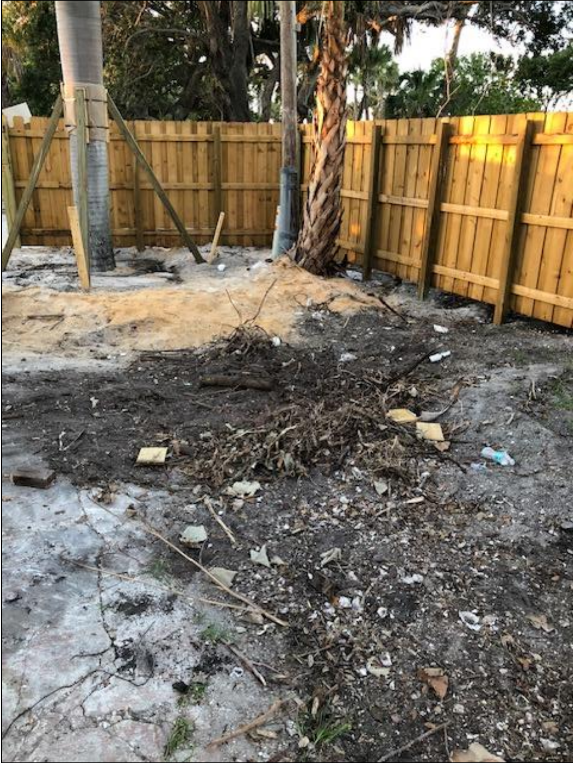
Figure 18. Post-fence installation and palm tree planting, facing south.
