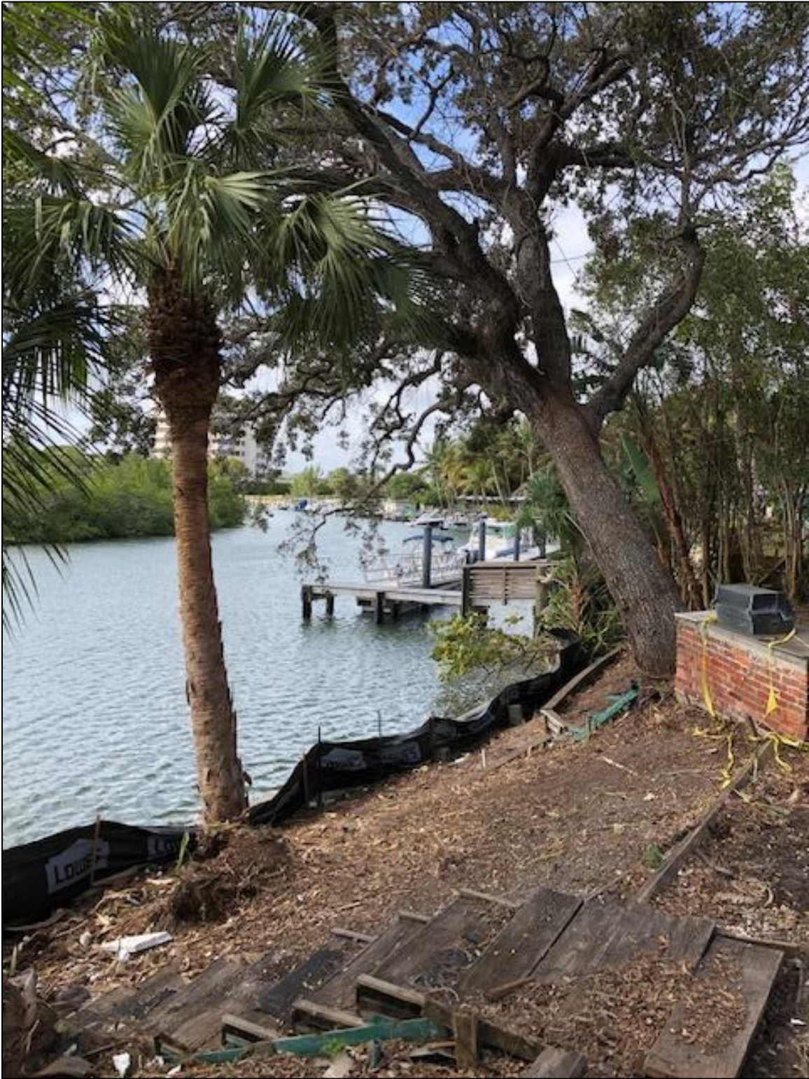
Figure 19. Pre-seawall removal and palm tree planting, facing northwest.
