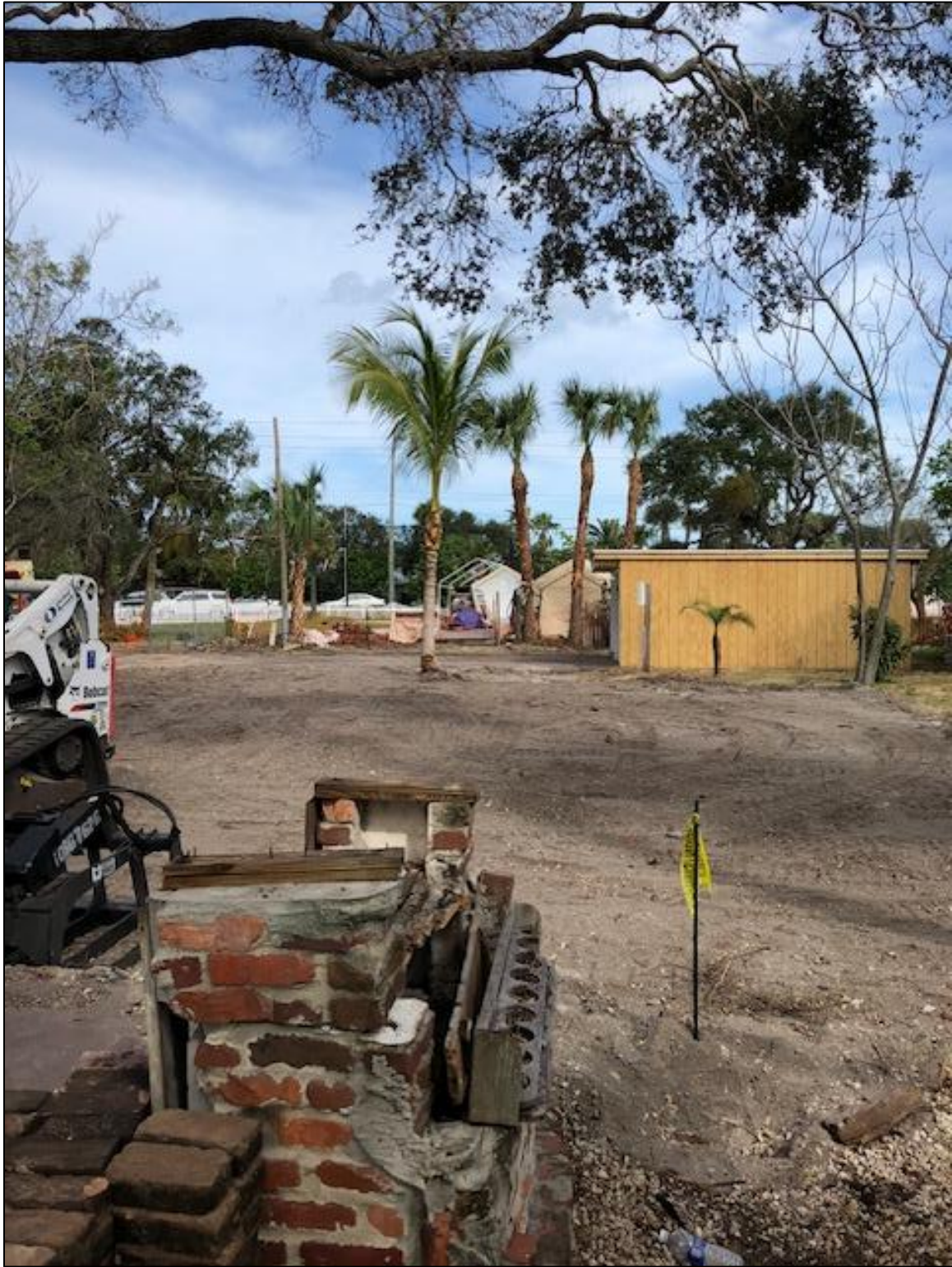
Figure 22. Post-fence installation, site dirt fill, and palm tree planting, facing south.
