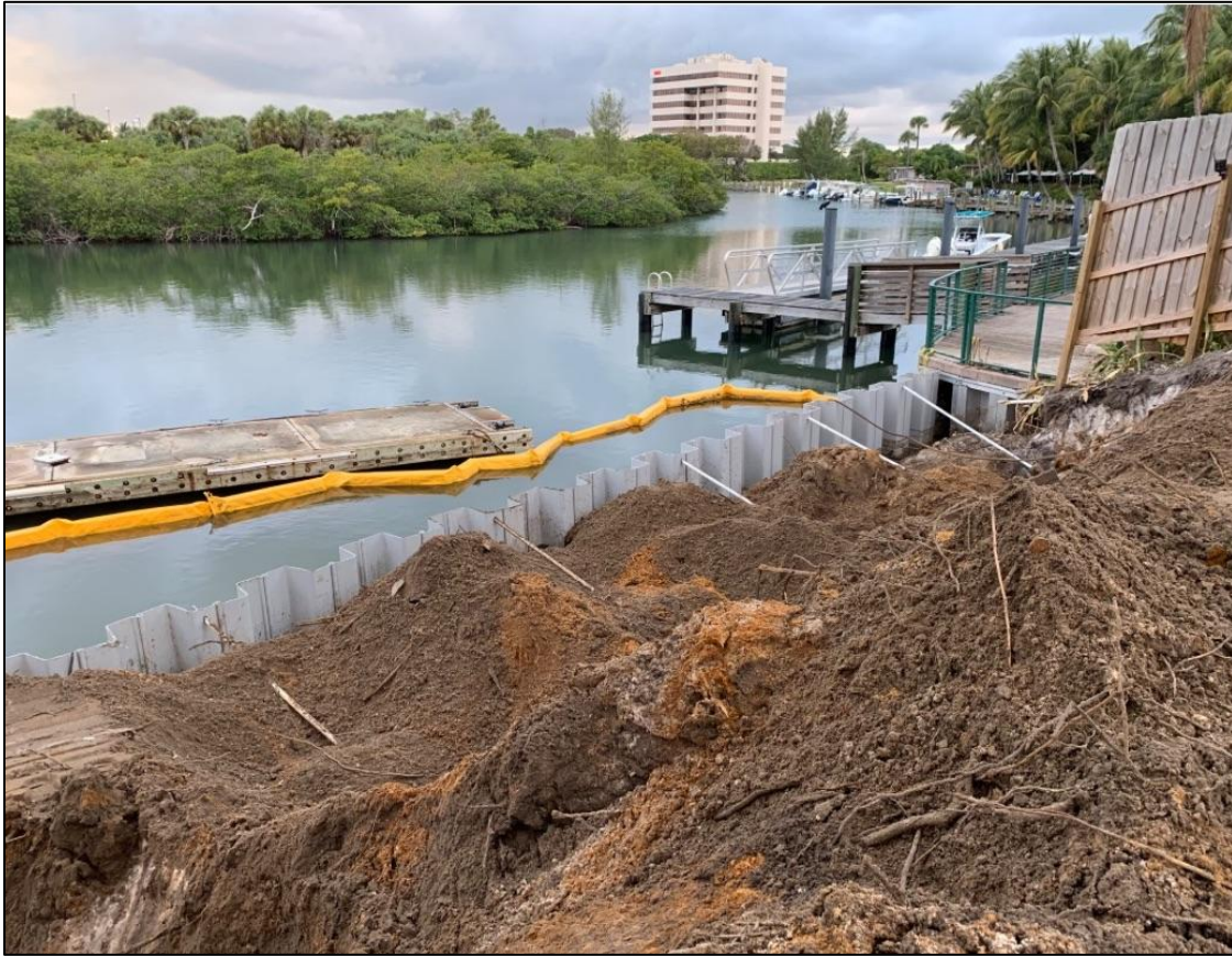
Figure 20. PA post-seawall removal and during new seawall construction, facing west-northwest.
