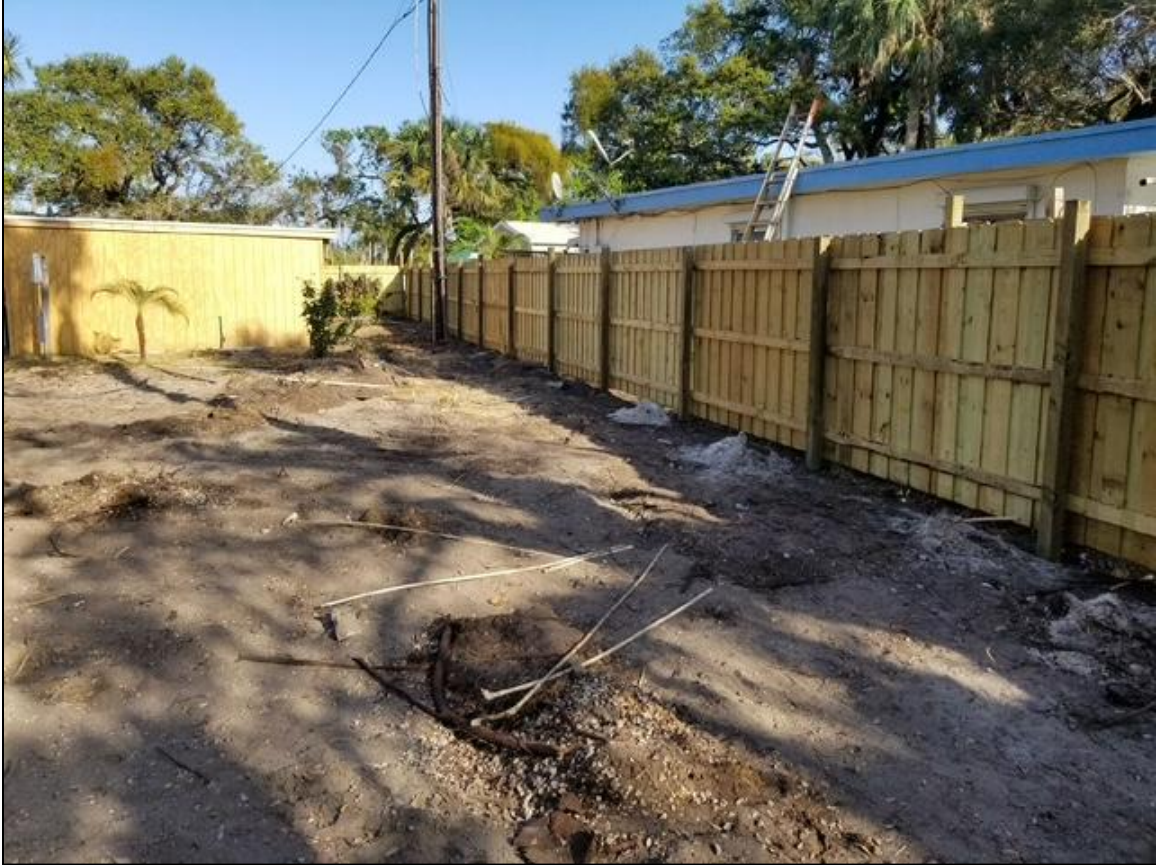
Figure 21. Post-site fill and fence installation, facing north-northwest.
