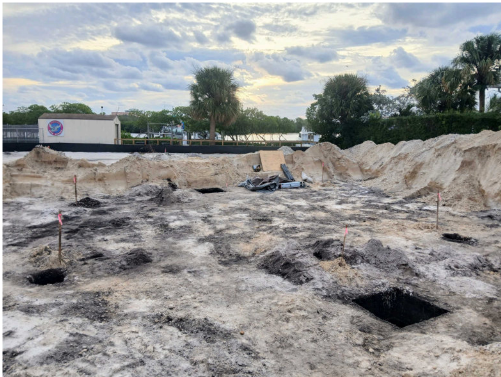
Figure 6. Above: commencing mechanical removal of fill from parcel, looking southwest.
