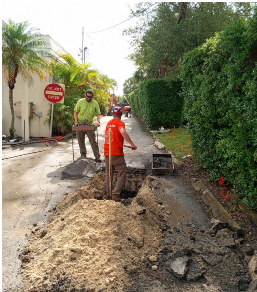
Figure 11. Sifting sediments from Shovel Test 2 within mechanically dug trench. Tests were dug counterclockwise around the building. View east along south side of structure.
