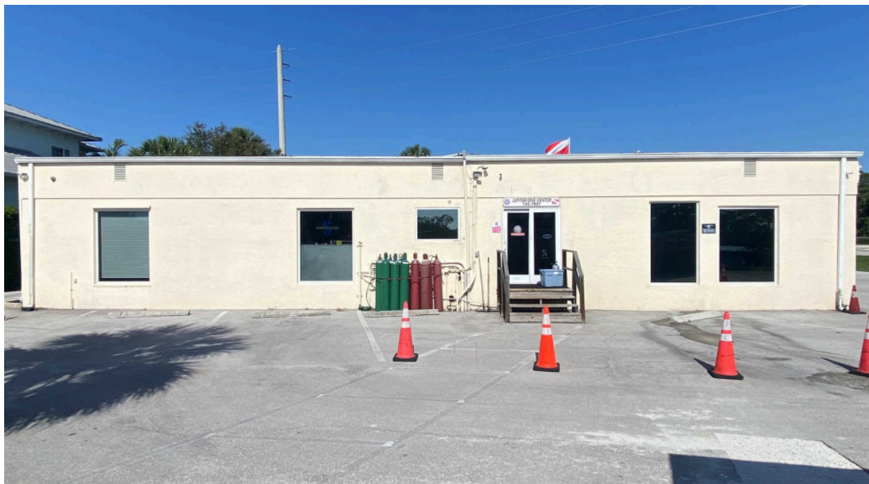
Rear of building looking west.
