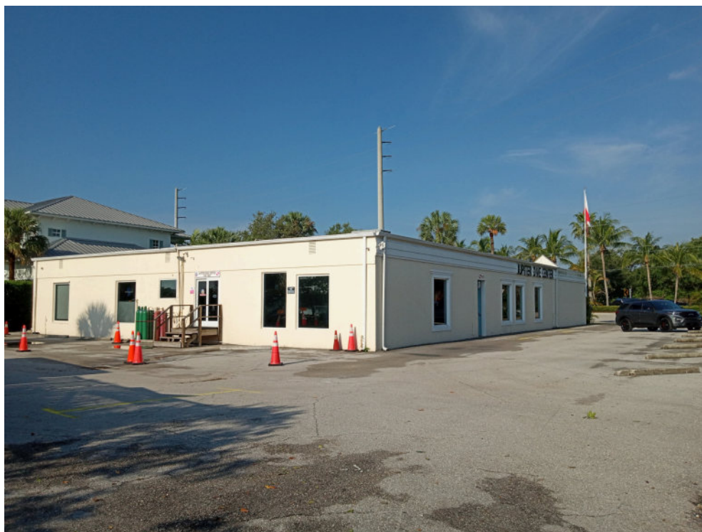
Figure 9. View of structure PB20324 looking southwest from waterfront.
