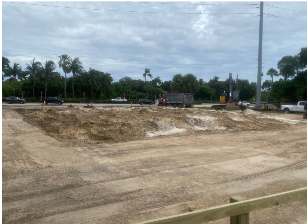
Figure 5. Project parcel with rear view of structure looking southwest in 2023 and after structure PB20324 was demolished in 2024.
