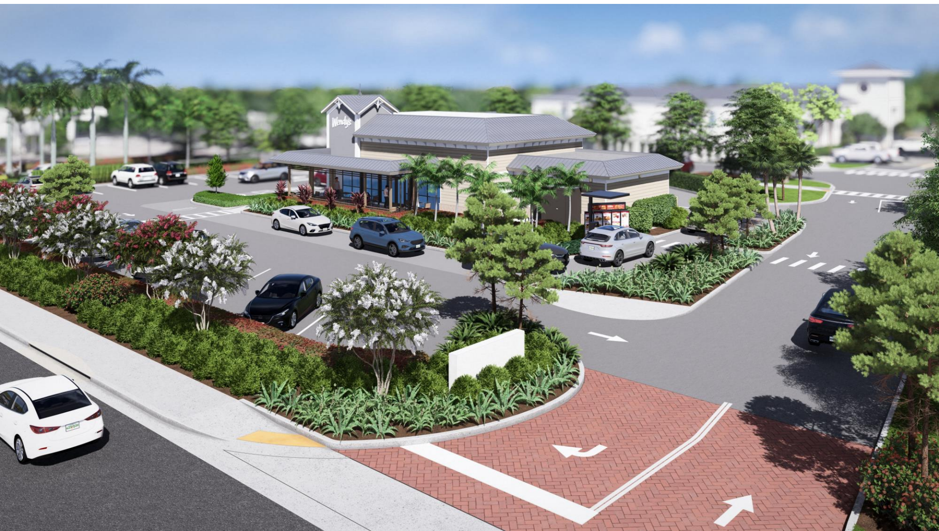
Aerial view looking into the site.
