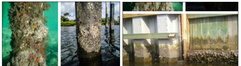
Figure 120 Pilings allow encrusting species to become established.
