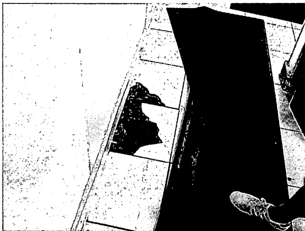
Missing tiles due to warping floor in kitchen/dishwashing building.
