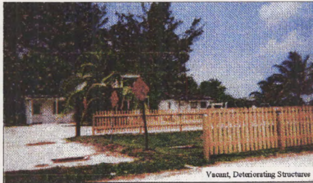
Vacant, Deteriorating Structures
