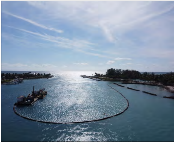
Figure 54 2023 Sand Trap Dredging Operation
