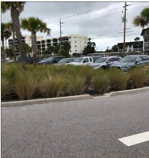
Figure 31 Bioswale mitigation for parking lot
