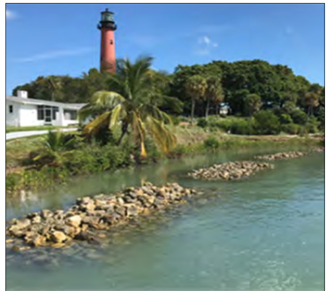
Figure 26 Shoreline protection via breakwater
