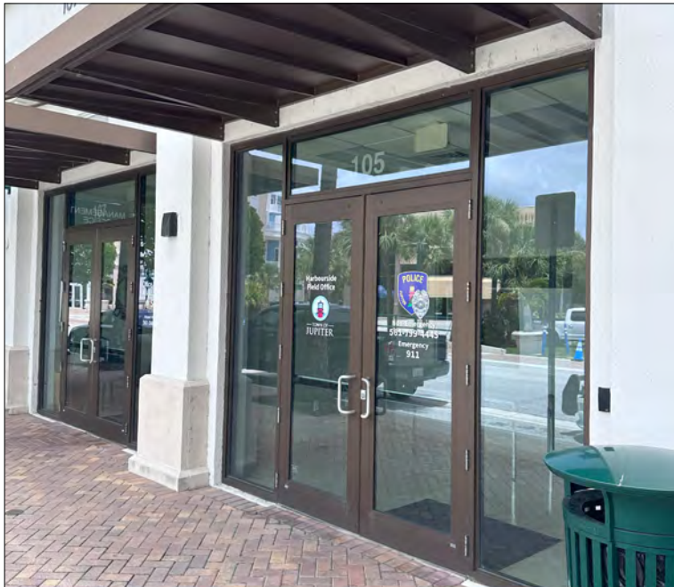
Figure 140 Harbourside Substation image.
