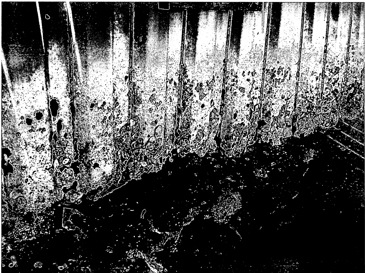
Metal Seawall showing significant corrosion including holes in the metal and several inches of at the bottom of the panels missing.
