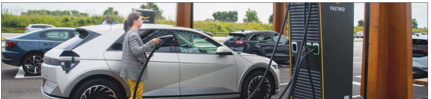
Figure 88 Examples above of electric vehicle charging infrastructure.
