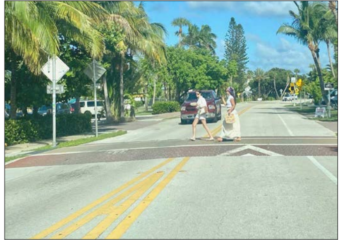
Figure 77 Raised crosswalk located along A1A near Guanabanas.
