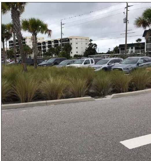
Figure 31 Bioswale mitigation for parking lot
