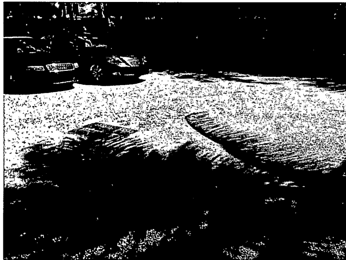
Valet drop-off area with gravel washed from around drain.
