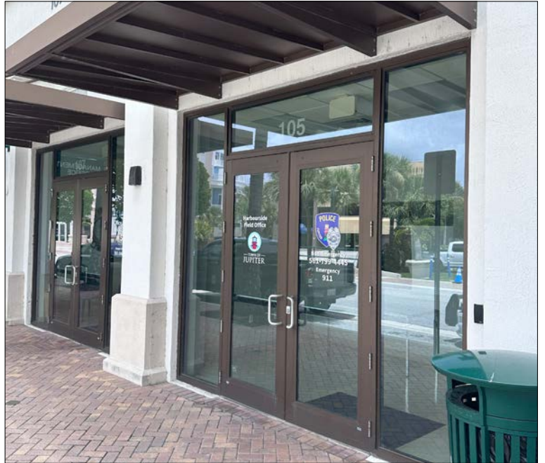
Figure 140 Harbourside Substation image.
