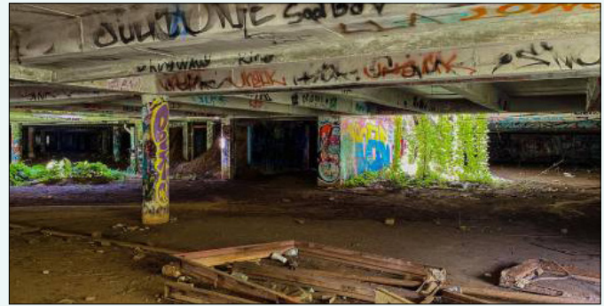
Figure 69 Existing conditions of Piatt Place
