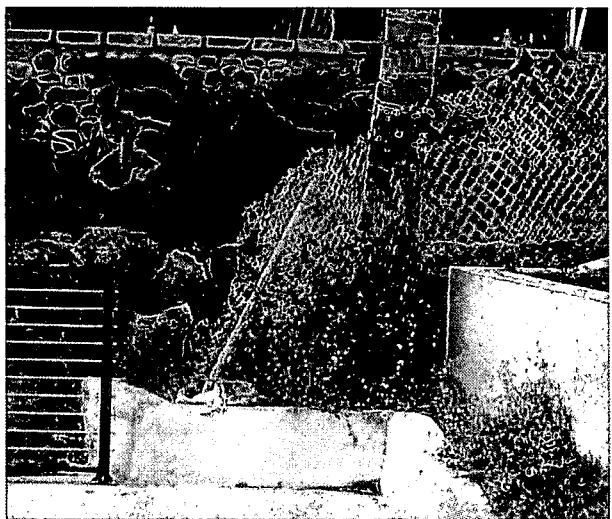
Inlet Village Marina fencing in disrepair
