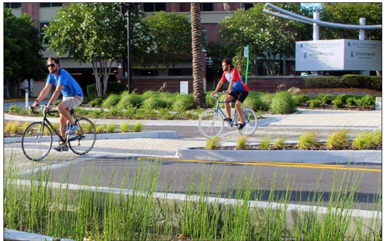
Figure 72 Example of a paved crosswalk and refuge.
