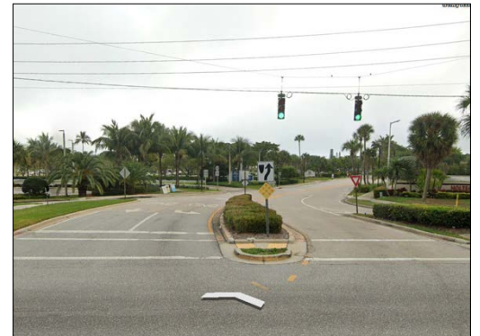
Figure 101 Entry into the CRA district at the US1/A1A intersection is a gateway opportunity
