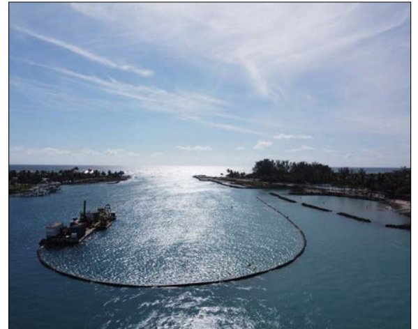
Figure 54 2023 Sand Trap Dredging Operation
