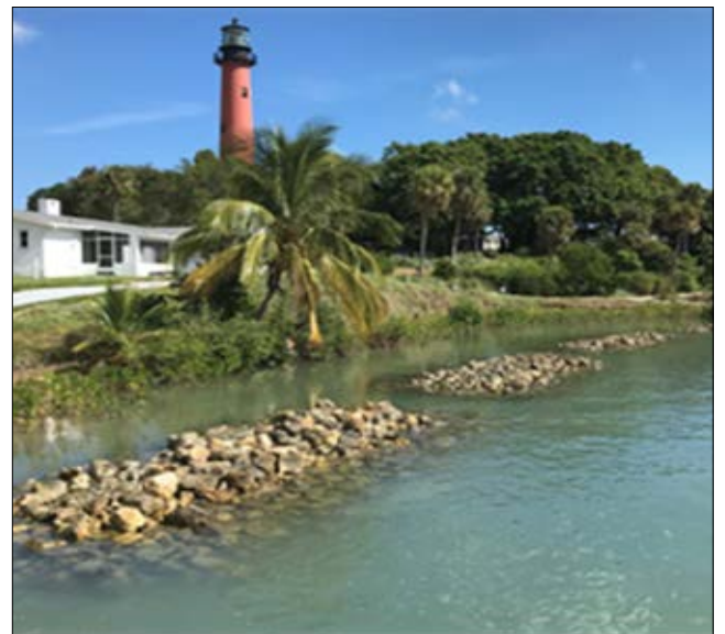
Figure 26 Shoreline protection via breakwater
