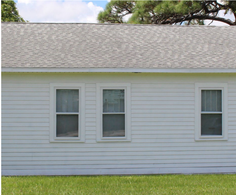
Figure 5: Photo of Existing Windows, East Elevation
