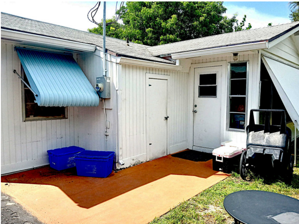
Figure 16. Rear entrance to 8PB20503 looking northwest.
