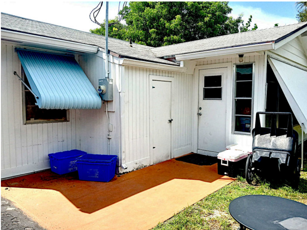
Figure 16. Rear entrance to 8PB20503 looking northwest.
