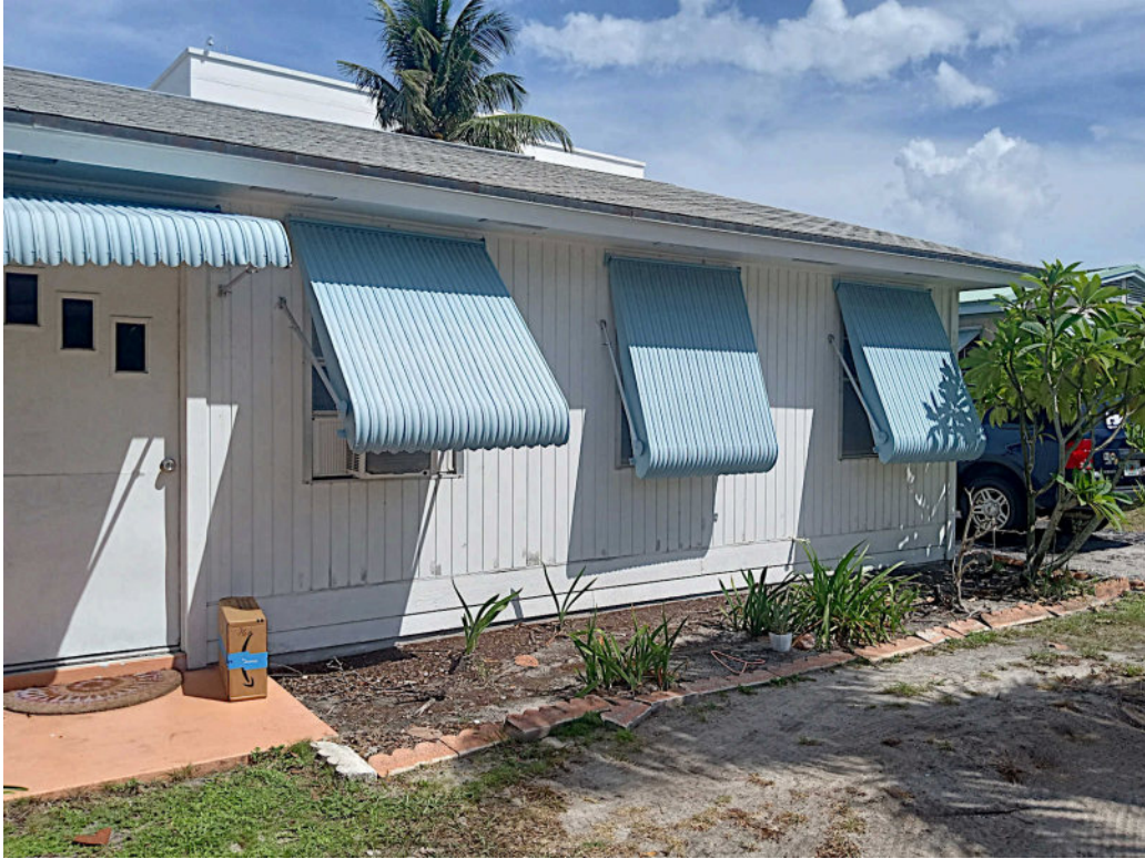
Figure 15. Main entrance of 8PB20503 looking southeast.
