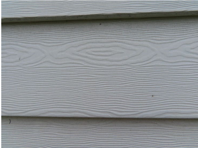
Figure 1: Photo of Existing Aluminum Siding
