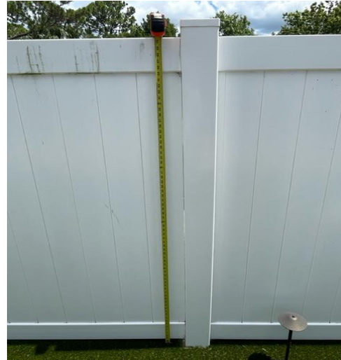
Interior of fence
