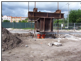
Field Load Test
