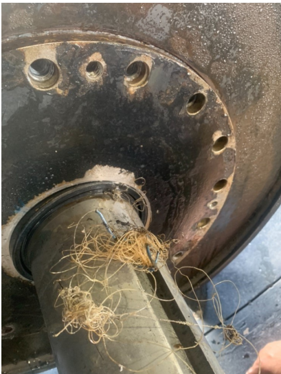
Fishing line destroyed oil seal
